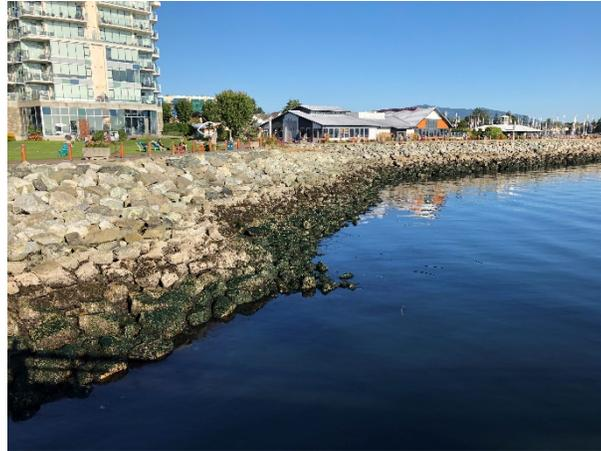
**Photo 1. Riprap breakwater found in the northern part of the project area.**
